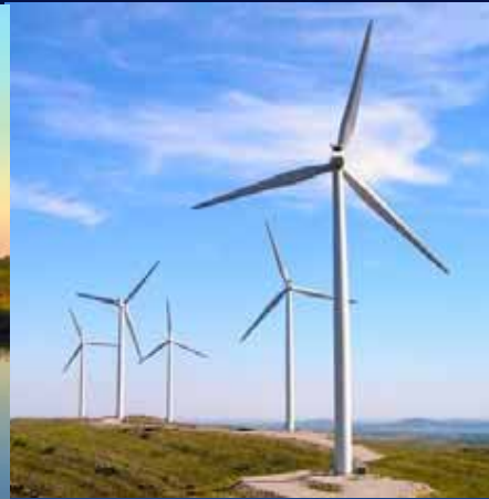
Blue Canyon Wind Farm 225 MW, near Lawton OK
